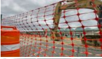
MacArthur Airport under construction
